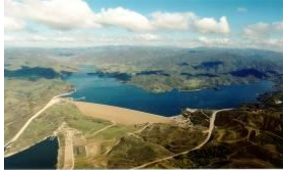
Castaic Main Lake and Lower Lagoon
